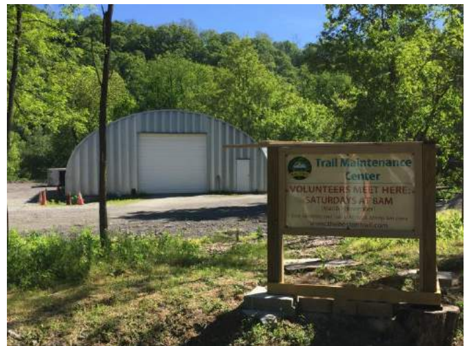
MYTC Maintenance Building
